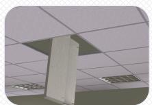
Pass cover diagonally through ceiling opening, or fold if the space is tight
