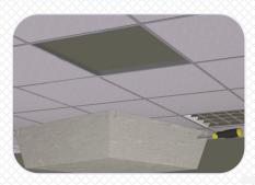
Pierce suitable holes in cover for cables to pass through. Note: cables should be a tight fit
